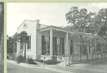
Office Building (H-E-B Visitor Center)
